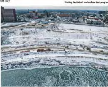
Starting the tieback anchor load test program
